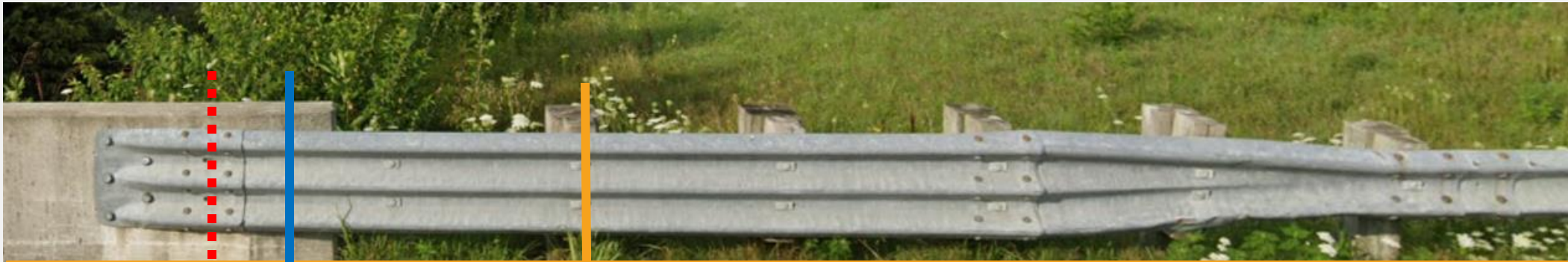
25'-0"-Limits of Guardrail Transition Type GB
