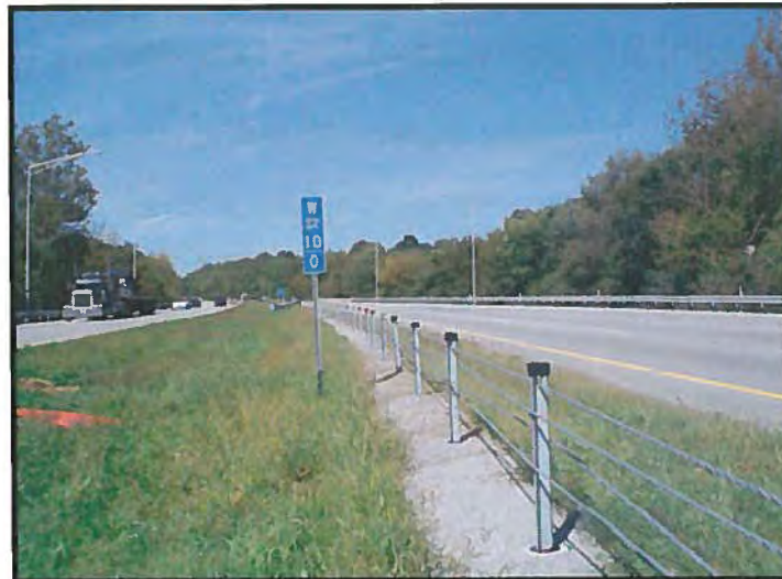
Completed Section of Brifen WRSF TL-4 (4-Rope)
