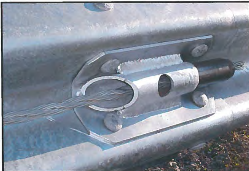
Attachment to Guardrail
