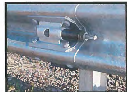
Picture 2.4 Attachment to Guardrail
