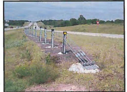
Wire Rope Gating Terminal (WRGT-FL)
