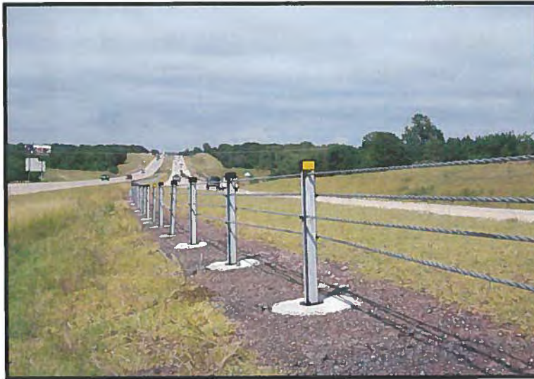
Completed Section of Brifen WRSF TL-4 (4-Rope)
