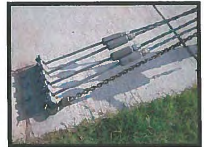
Picture 4.17 Come-Along Hooked to Side of Anchor Frame
