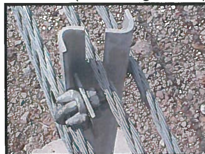
Temporarily Clamp the Rope
