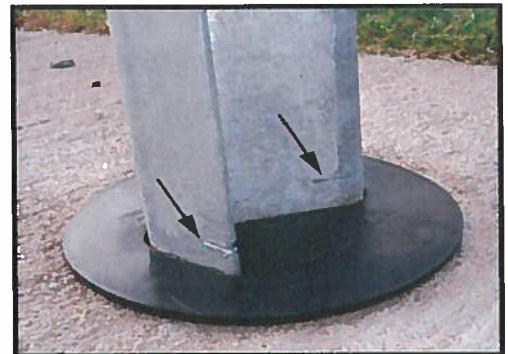
Weakening Cuts (Toward Anchor)
