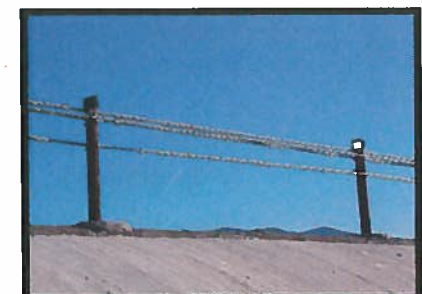
Completed Section of Brifen WRSF
