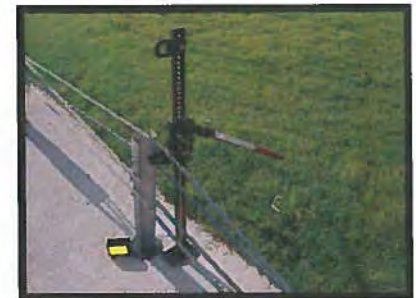
Picture 4.18 Hi-Lift Jack Raising Ropes
