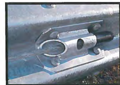
Picture 2.5 Attachment to Guardrail
