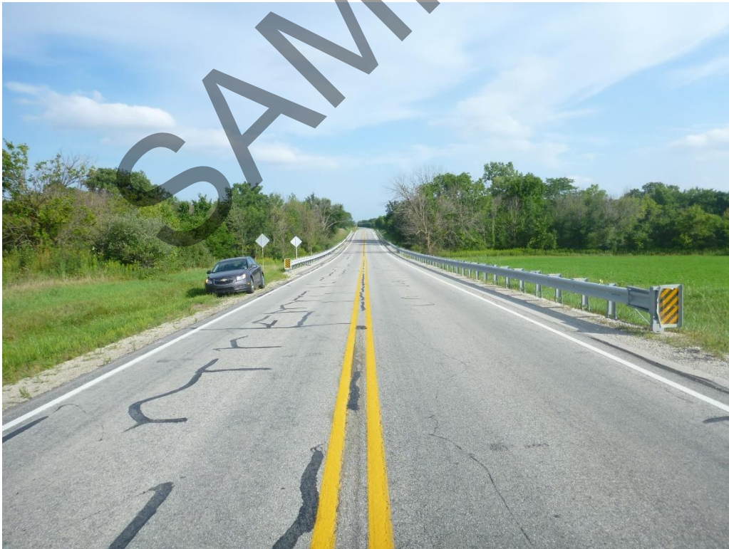
Northwest Approach to Structure - Looking Southeast
