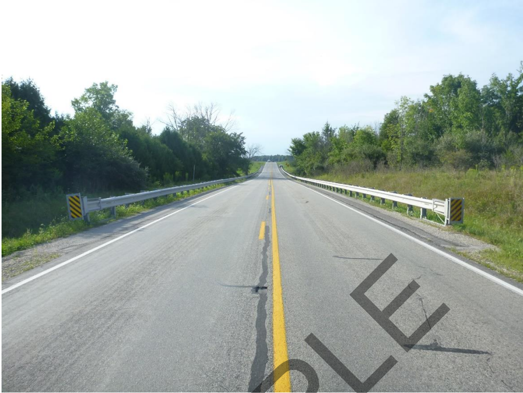
Southeast Approach to Structure - Looking Northwest
