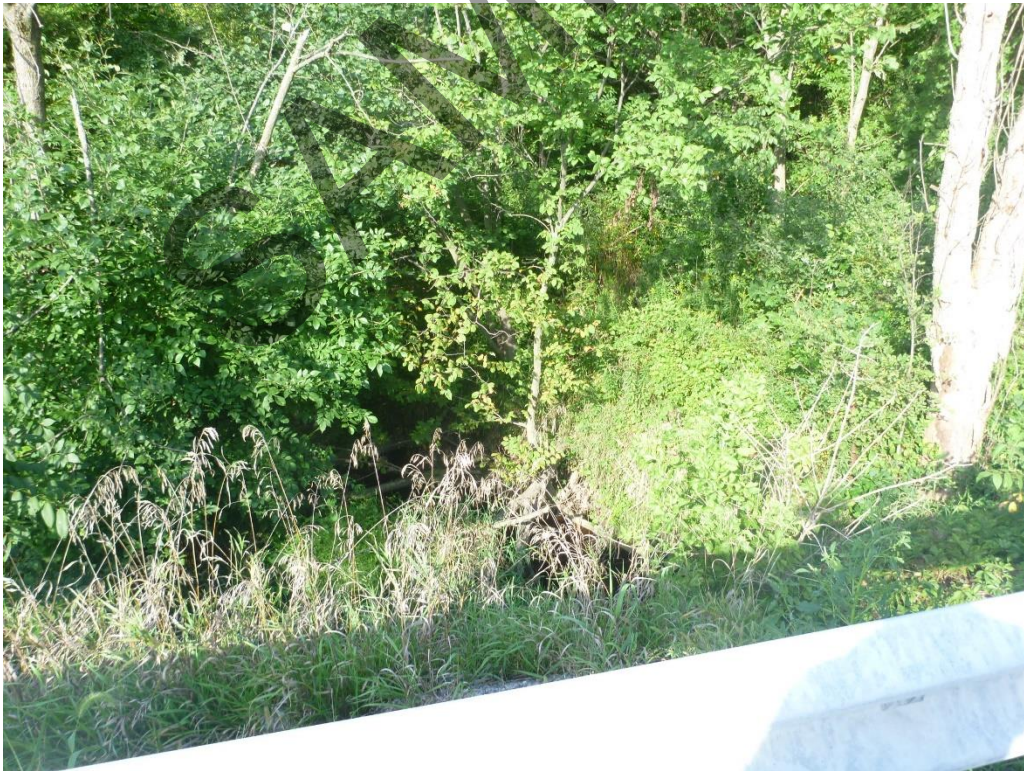
Looking Downstream (Northeast) from Structure
