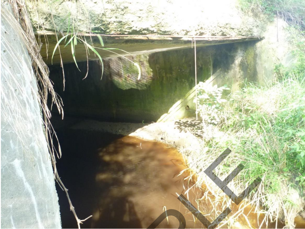
Southwest (Upstream) Face of Structure - Looking East
