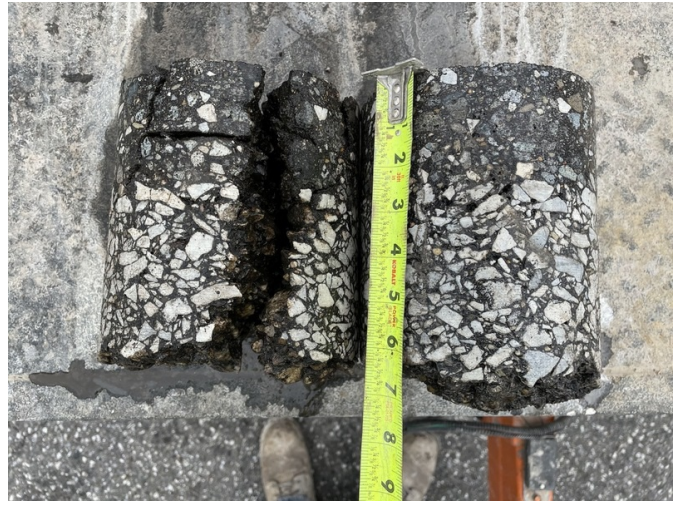
Pavement Samples taken during Investigative Sampling
