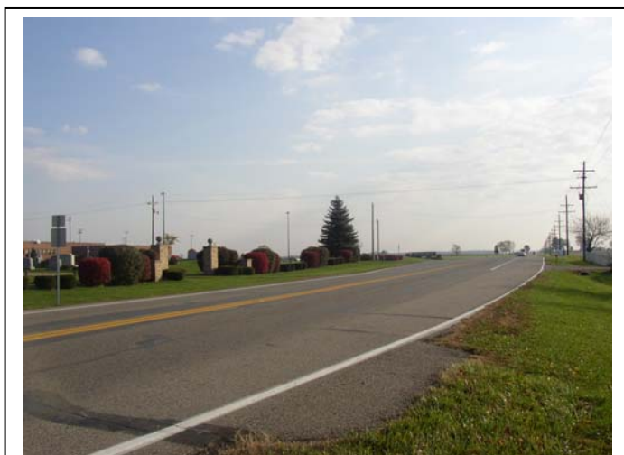
SR 32 is a rural two-lane highway with narrow shoulders through most of Boone County.
