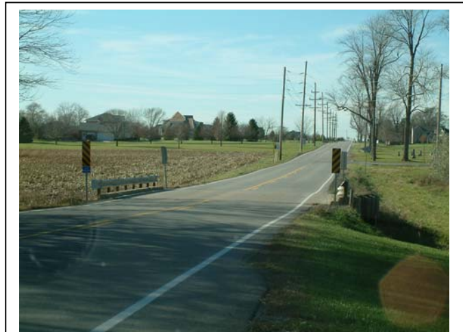
SR 38 is a two-lane, rural roadway with narrow shoulders through Madison County, except within the Town of Pendleton
