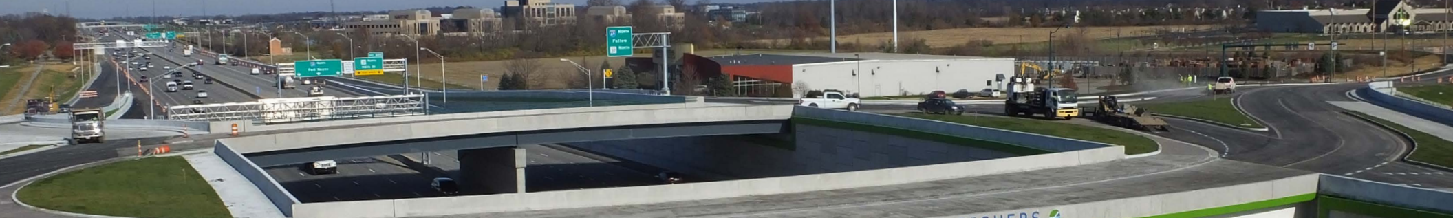
Interstate 69 at East 106th Street, Fishers, Indiana
